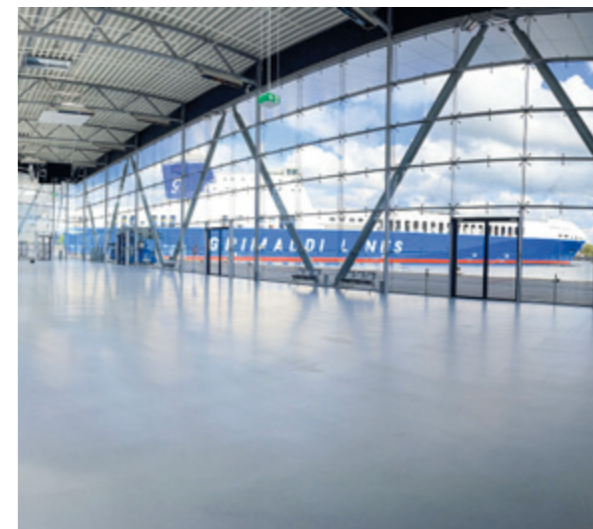
EMERGENCY COMMUNICATION Cruise terminal, Rostock Port
