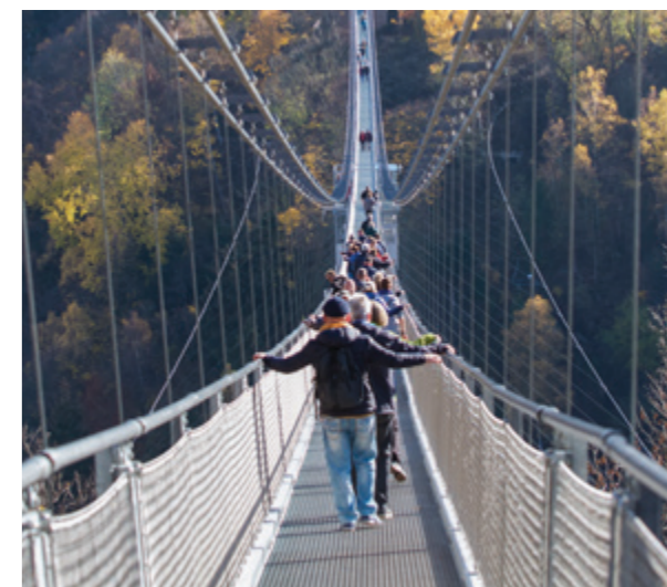
OUTDOOR SOUND SYSTEM Harzdrenalin steel bridge
